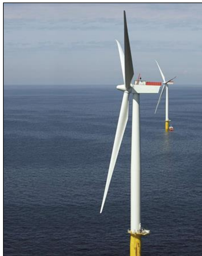
Figure 3.2 Wind turbines at Walney offshore wind farm.
