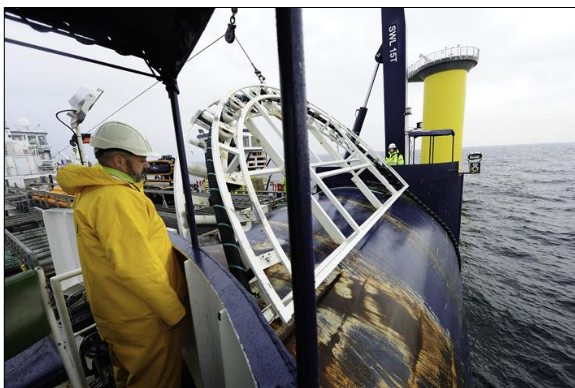
Figure 3.7 Array cable installation at the Gode Wind offshore wind farm.
