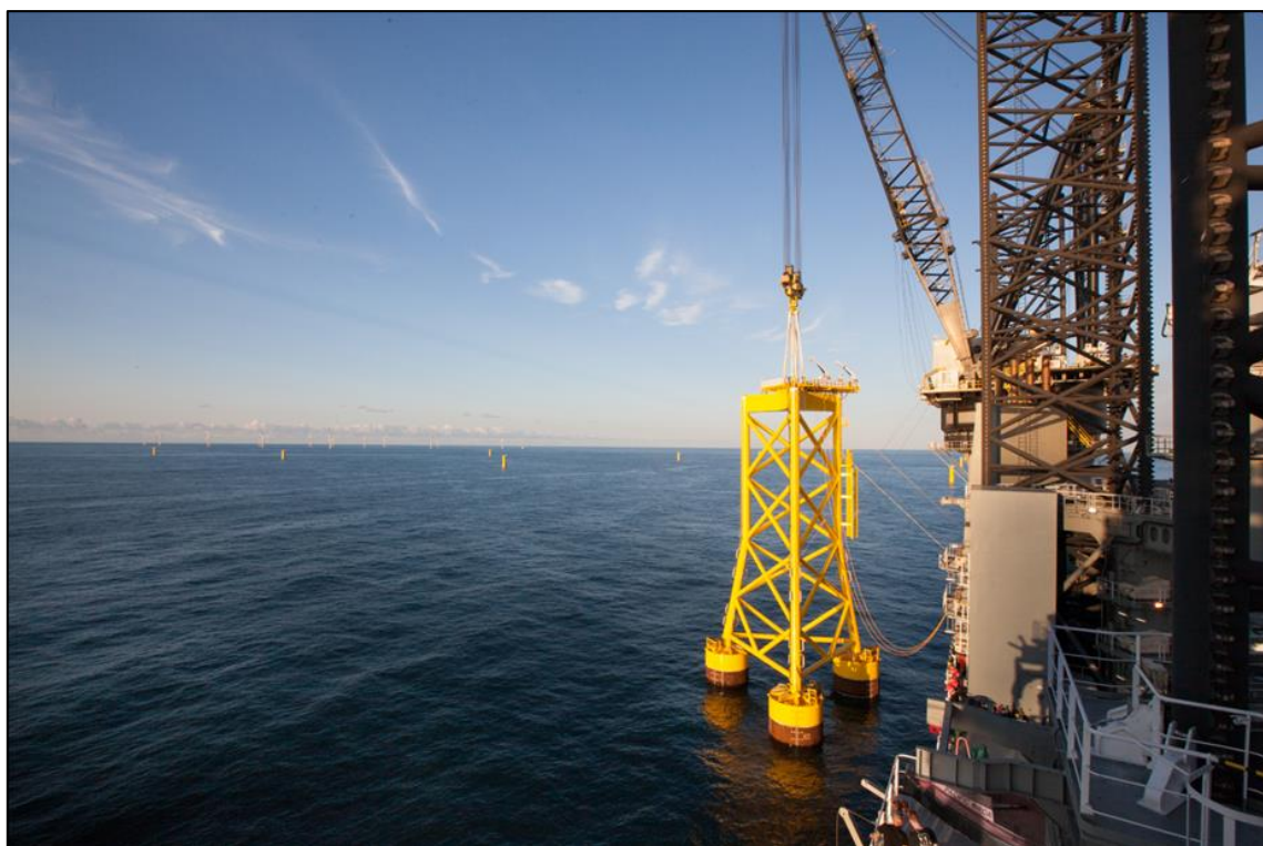
Figure 3.4 A jacket foundation with suction buckets being installed at the Borkum Riffgrund One offshore wind farm.
