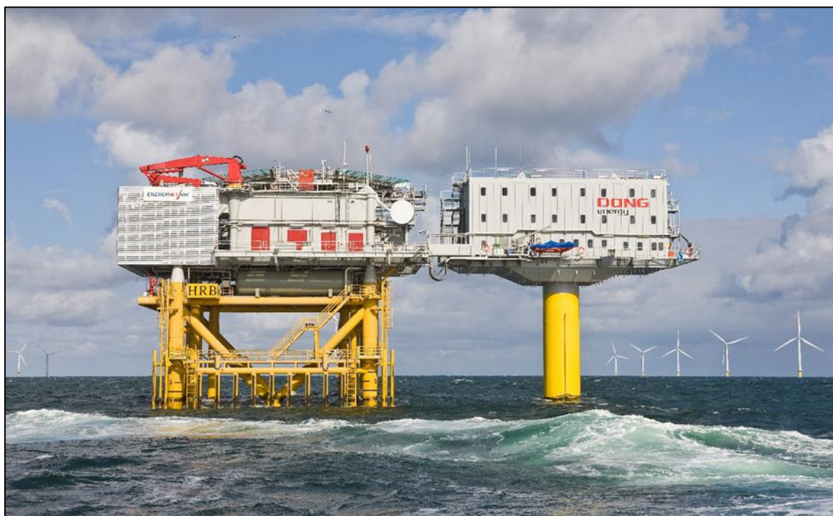
Figure 3.8 Offshore accommodation platform (right) at the Horns Rev 2 offshore wind farm, sited next to an offshore substation (left)*.
